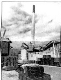
The average worker at the Elmore plant makes $18 an hour — a solid amount in a farming community with few factory jobs.
