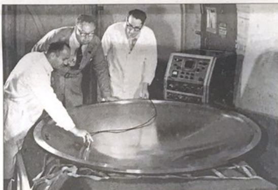
Beryllium was an essential metal during the Cold War. Among the uses: heat shields (above) for the Mercury manned flight program.
